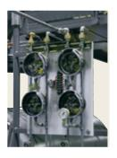
Electrical Controls - Electrical controls include a weather-proof panel with a main disconnect switch, individual motor starters, and disconnect switches
