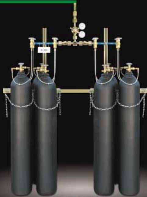
Oxygen Manifold
